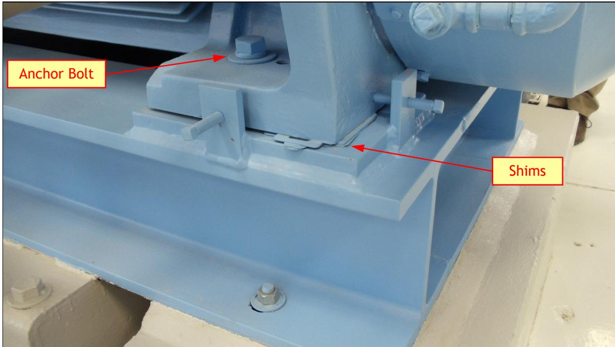
Fig. 4: How not to shim a machine
